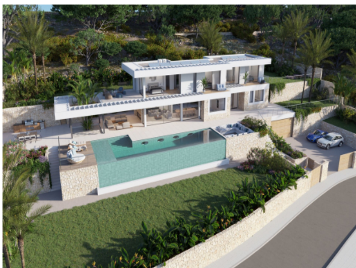
View on the project
