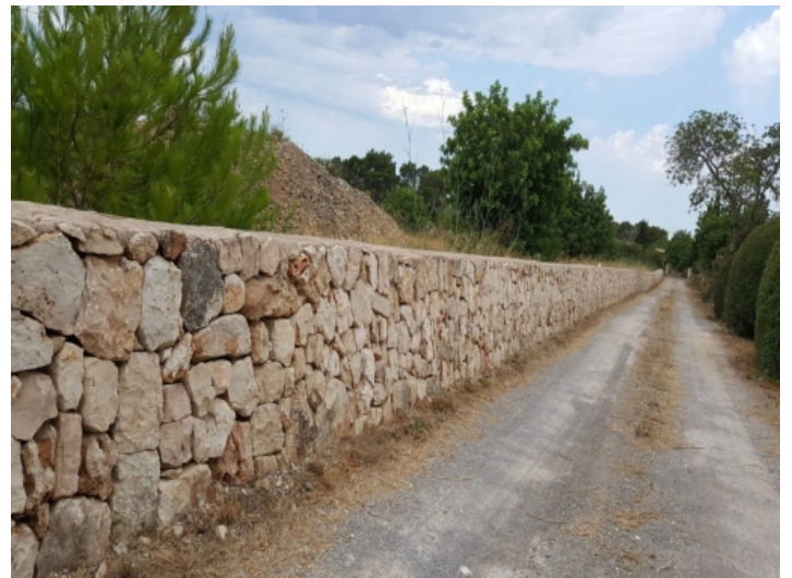
There are newly-built Mallorcan walls
