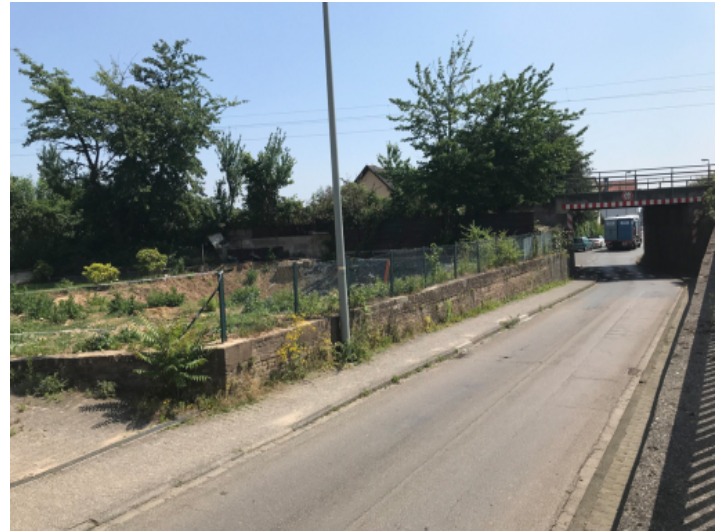
Views to the tunnel
