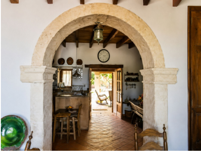
Historic Stone Arch in the Main House
