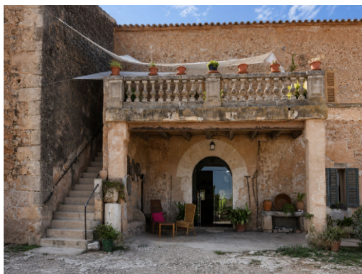
Main Façade with Terrace
