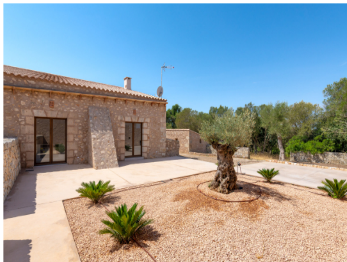
Terrace with access to the kitchen and living room
