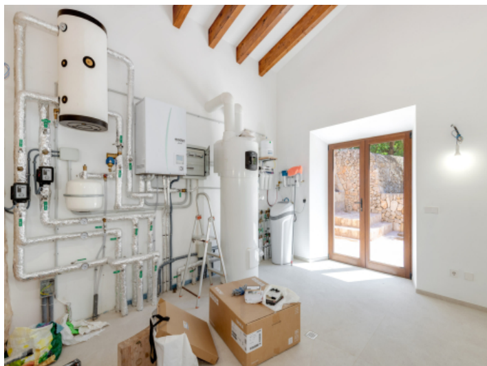
Storage and utility room
