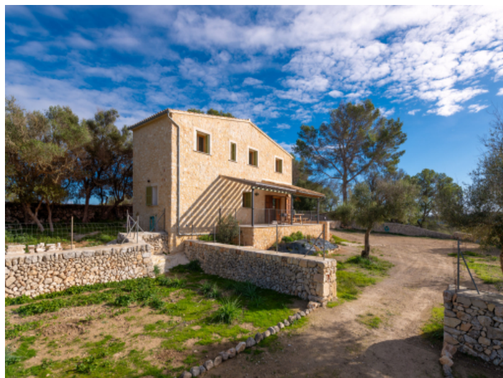
Exterior view of the finca with covered terrace
