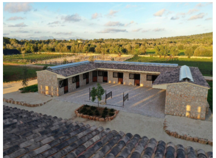
One of five stables with forecourt
