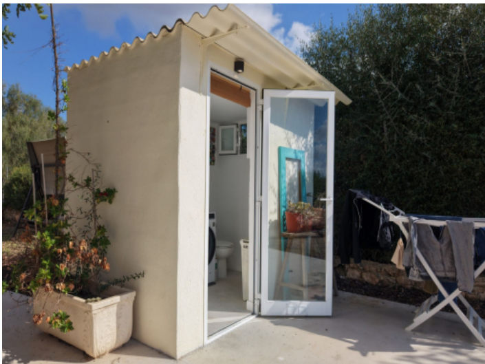
Laundry room and WC
