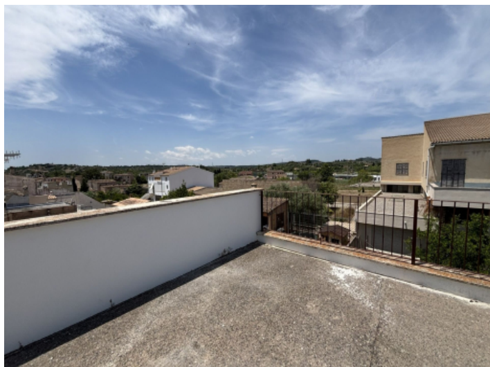
Spacious and sunny rooftop terrace
