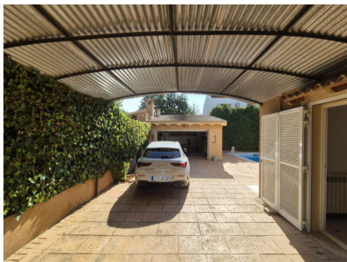
Garage and carport
