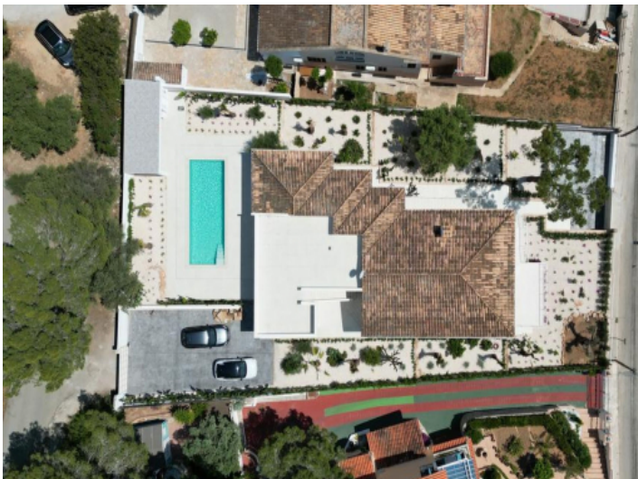
Aerial view of the villa
