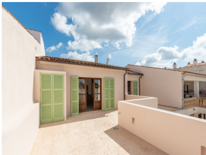
Terrace on the first floor
