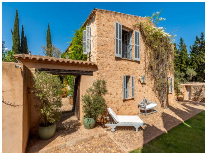
Facade of a typical mallorcan country home
