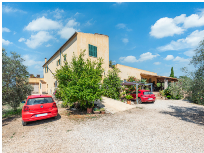
Access to the house
