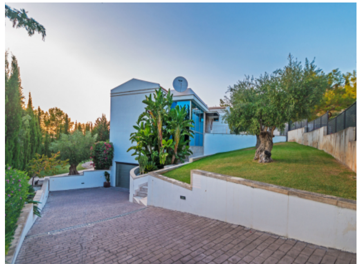
Large driveway to the garage
