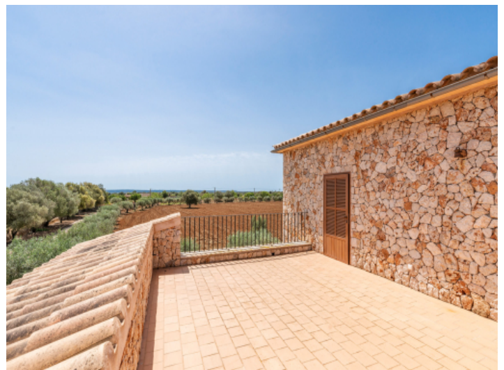
Upper terrace with a view
