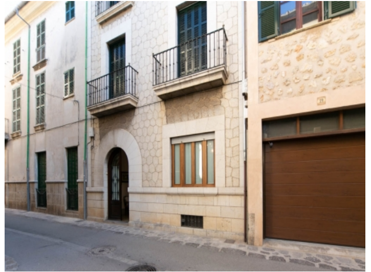
Exterior view of the town house
