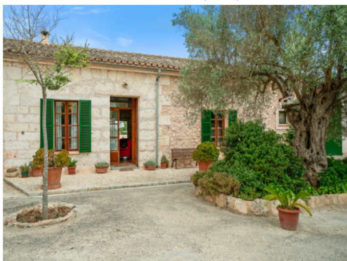
Access to the house
