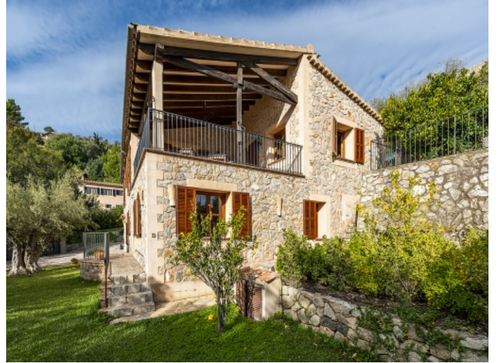
Exterior view of the stone finca
