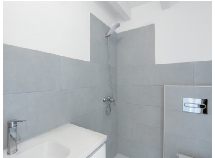
Bathroom with shower
