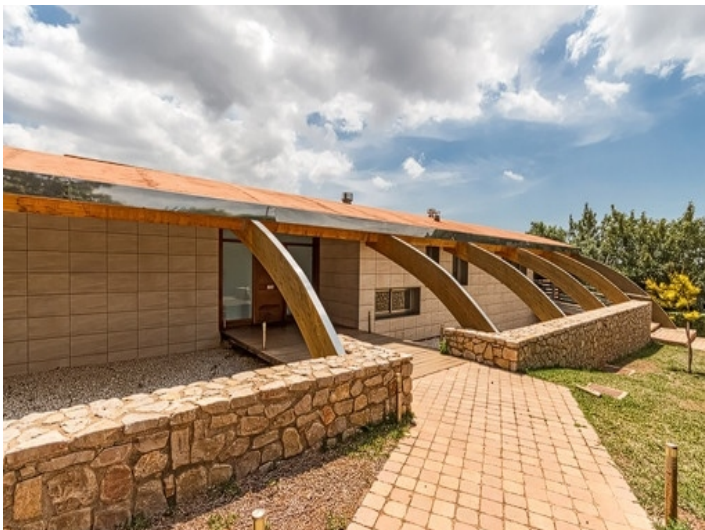
Interestingly designed entrance
