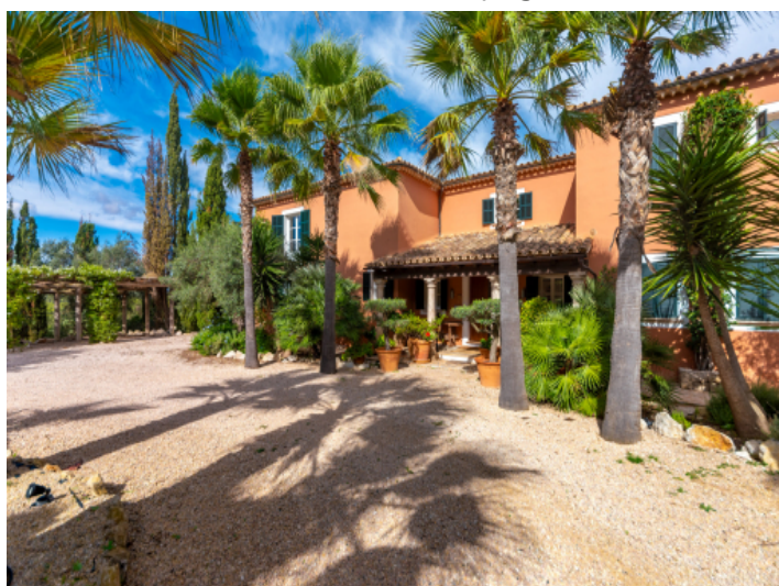
Exterior view and main entrance
