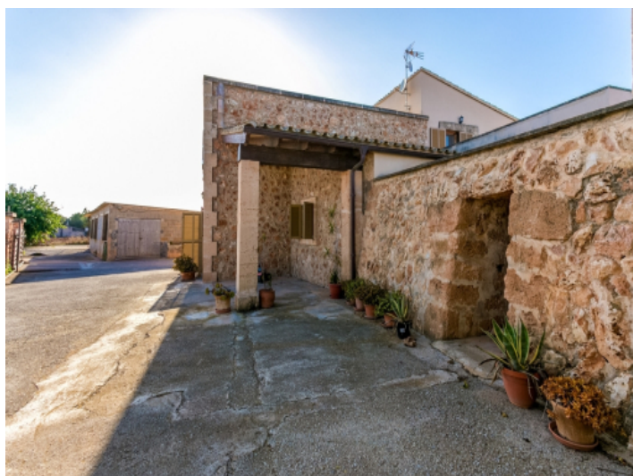
Typical natural stone walls
