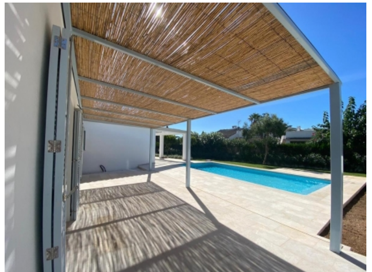
Covered terrace of the villa
