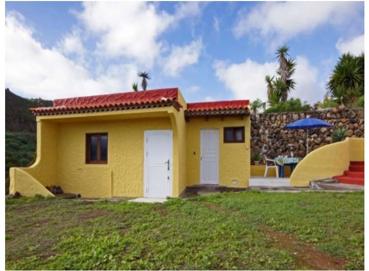
Separate house for guests, storage, office, etc., with practical outside bathroom
