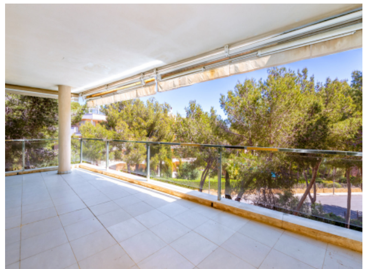
Covered terrace on the living level
