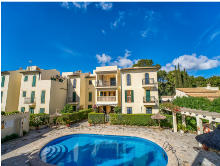
Complex and pool area
