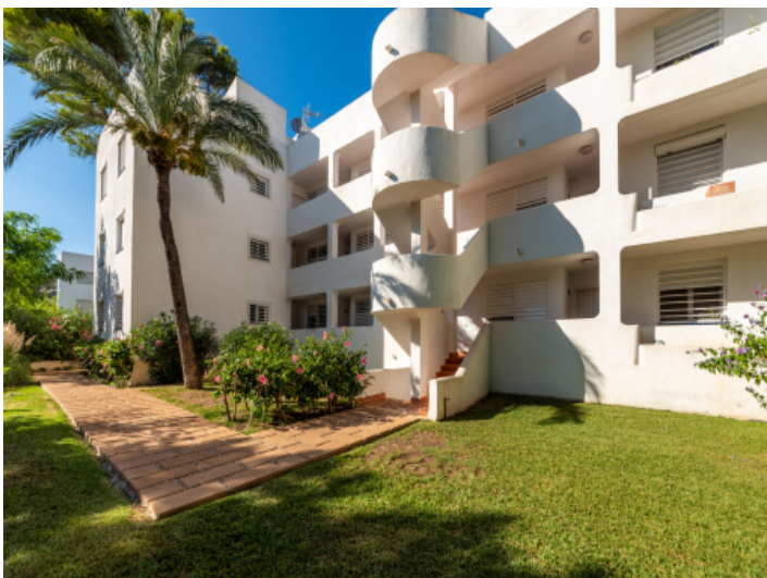
View of the building
